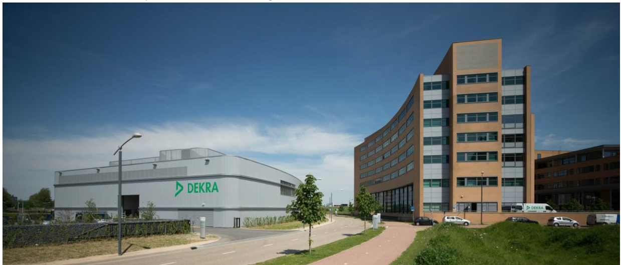
The DEKRA laboratory and office building
